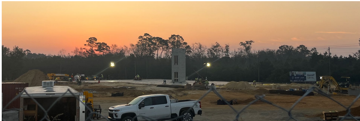
Drone and Multivista being used to document the project.
